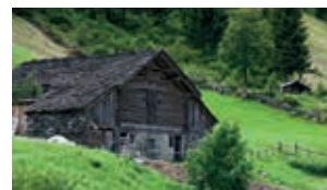
Typical barn with hayloft in Val Corta
